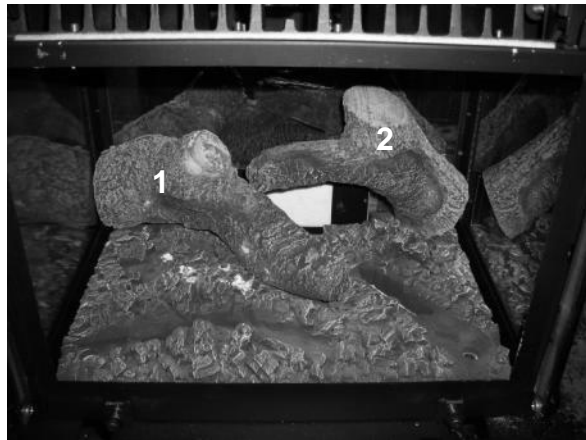
Figure 32 – Log 2 in Position
