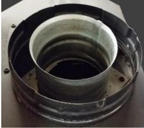
Vent Attachment Inspection – unbent and attached rings
