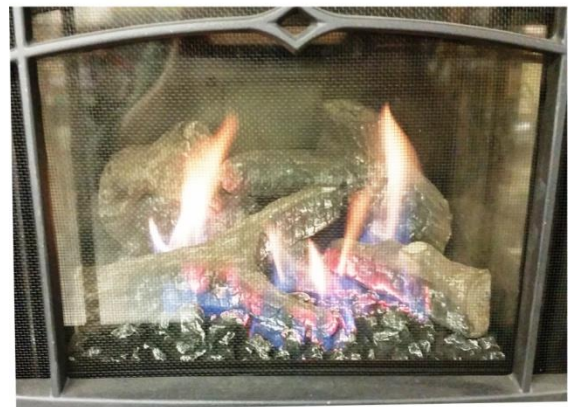
Figure 40 – Typical Burner Flame Appearance
