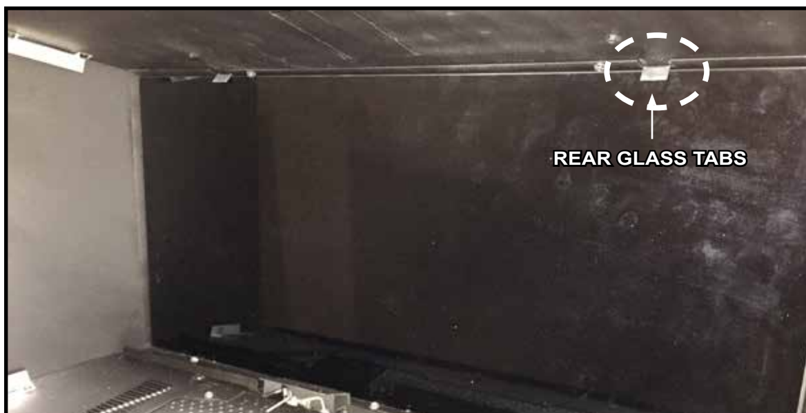
Figure 5 Install Rear Glass Panel
