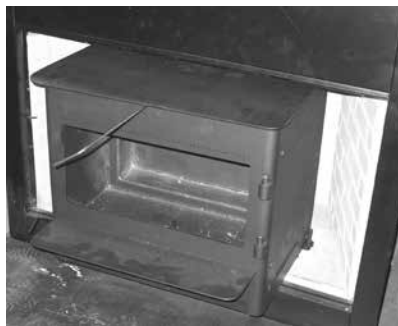
Pull Rod in place Diagram 6
