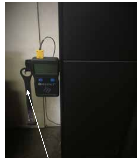
Air and Bypass operating handle/monitor storage.
