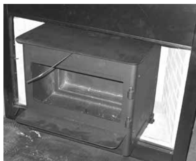
Diagram 5 Pull Rod In Place
