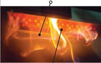
Bypass closed; located inside firebox (top front)
