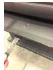
Air control for heat output
